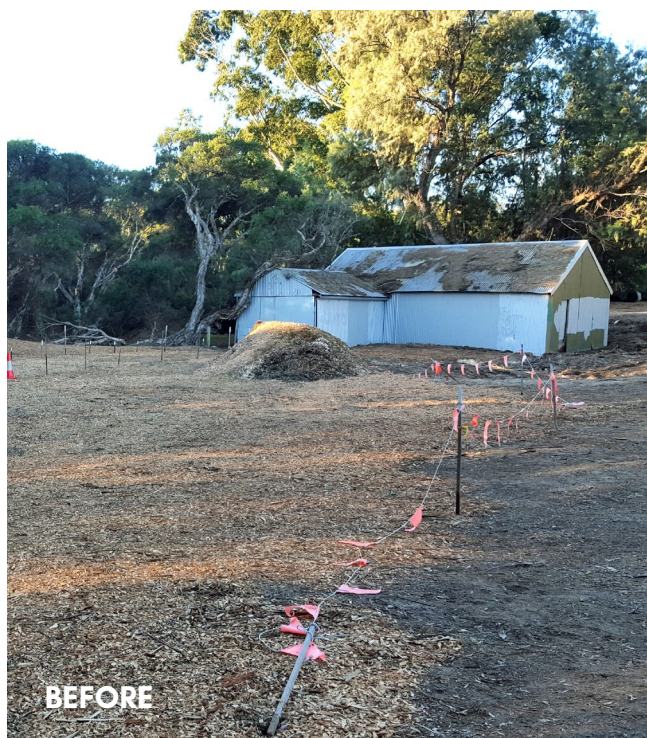
FOLC meeting shed before planting and painting. Photo: Naga Srinivas
